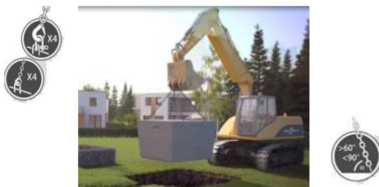
Fig-16: Manutention de cuve
